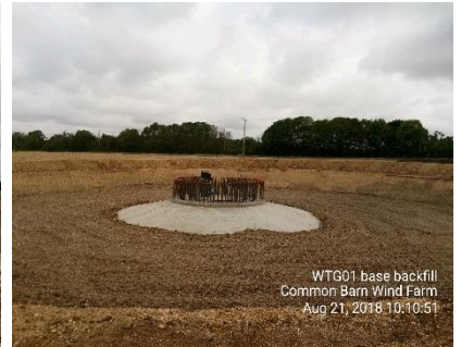
Partially backfilled foundation
