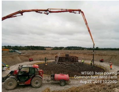
Pumping concrete into foundation
