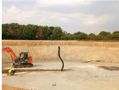
Cable duct installation
