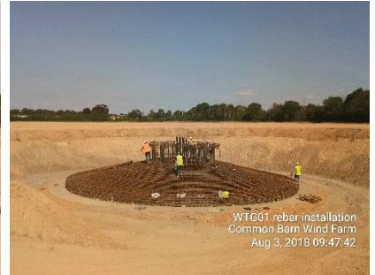
Fixing reinforcing steel ("rebar")
