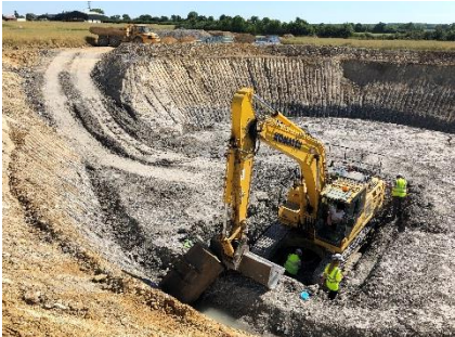
Testing of foundation formation
