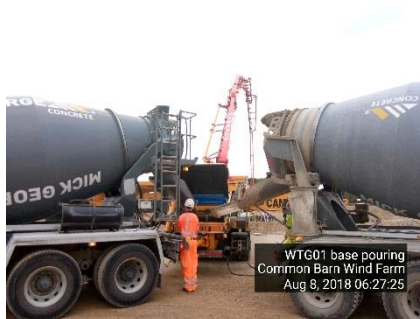
Discharging concrete into pump
